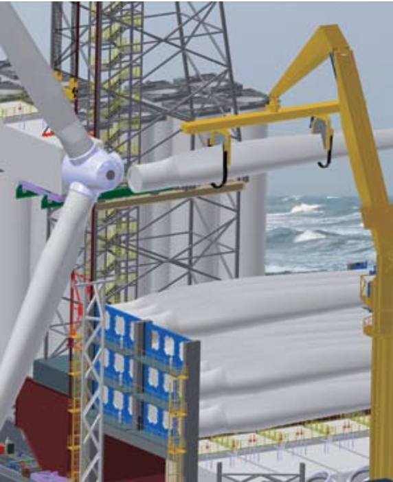
Image 3: The blade is picked up by a Knuckle Boom Crane with a dedicated gripper
