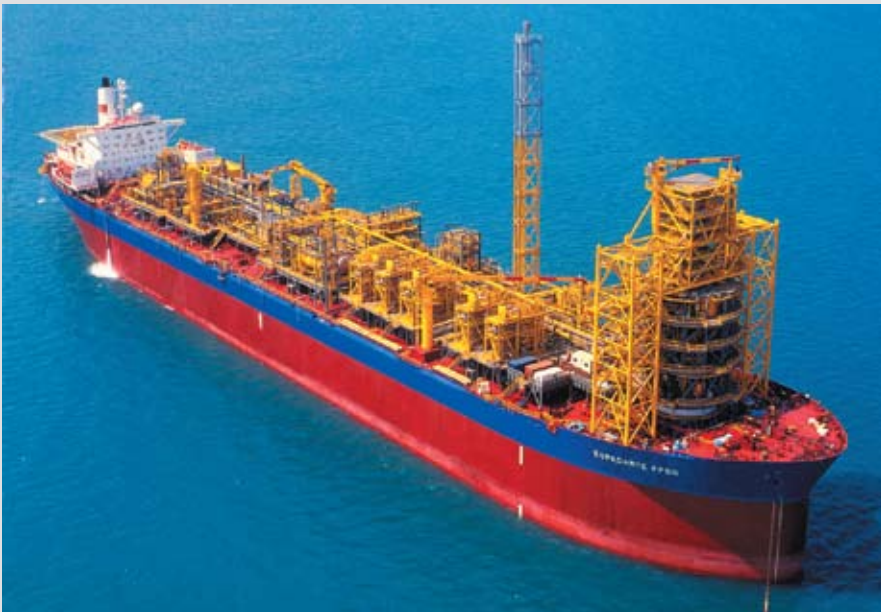
First converted by Keppel Shipyard in 2000 for SBM, FPSO Espadarte will return to Keppel Shipyard for an upgrade
